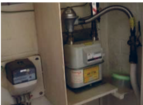
Asbestos panelling around a gas meter
