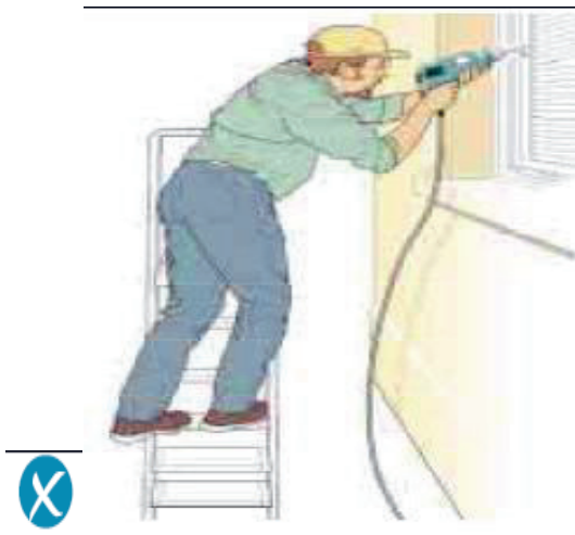
Incorrect – steps side on to work activity
