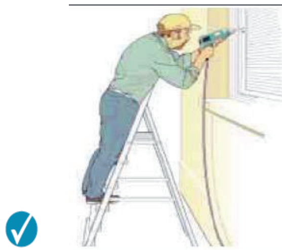
Correct – steps facing work activity
