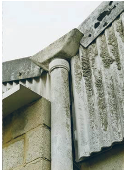
Asbestos cement downpipe, hopper and profile sheet
