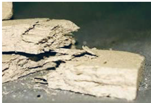
Pieces of Asbestos Insulating Board (AIB)
